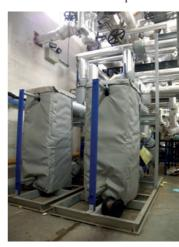
exchangers pre-boost the heating and the hot water so we don't have to use as much steam. It's boosting the water that's going into the calorifiers, which are now over 30 years old.
